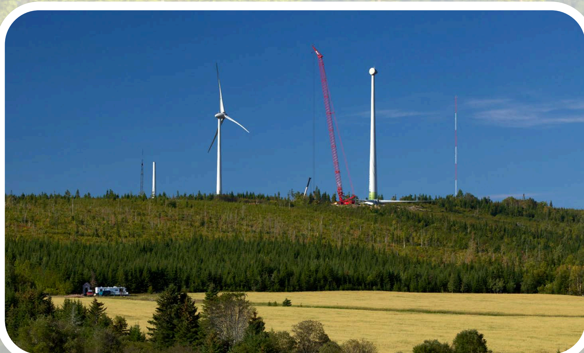
Tower installation des tours
